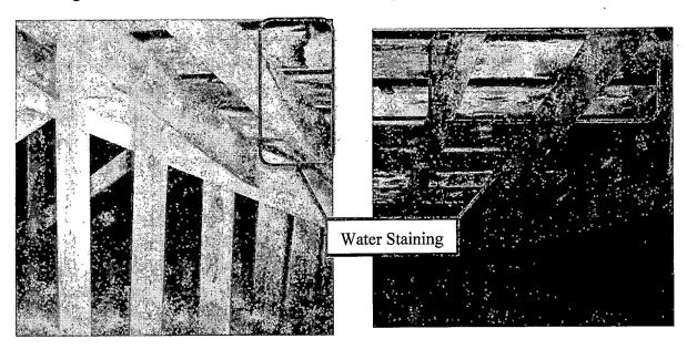
The same conditions observed in the south-east attic are expected to be found at roof framing throughout the rest of the building. Coordination with the tenant is needed to verify the expected condition of the framing in other attic areas. Although these areas were not accessible, the presence of water-damaged ceiling tile throughout the building is visible from inside the building and indicates ongoing roof leakage issues.
