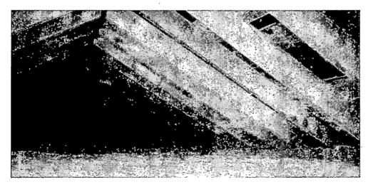
This attic area had multiple locations that indicated water had leaked through the shingles to the roof framing. The condition of the 2x6 roof framing, although not analyzed or tested, appeared to be adequate. No sagging or dry rot was observed. It appeared that little-to-no
